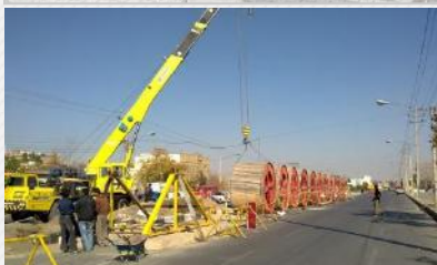
Cabling of 132 KV Transmission Line of Sepad and Bou-Ali Posts
