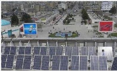
Purchase & construction of 240 kw SOLAR plant
