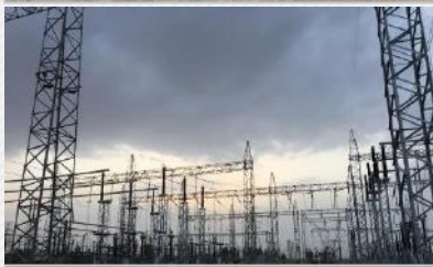
Providing ground station and ground system and complete executive operations for 400 KV line from Shadmehr to Torbat Jam (Phase 2)
