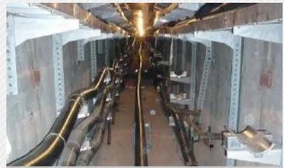
Installation of Cable Supporting Accessories and 230 KV cabling of xlpe Post of Azadegan to Ghourkhaneh
