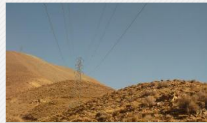
Supplying and installing 63 KV from Zahedan to Kourin;
