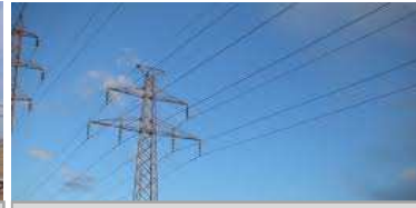
Procurement of supply and design of 132 KV transmission line from Tabas to Deyhuk
